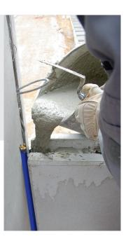
Joint is filled with plastic joint filling mortar
