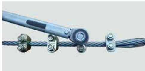
Fig. 12: Tightening of the collar nuts with a torque wrench
