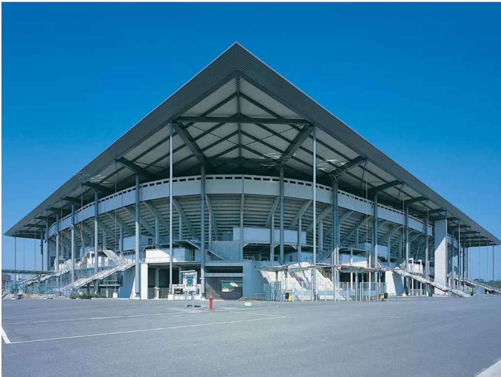
1 Ring cable with lower radial cables and upper steel girders
