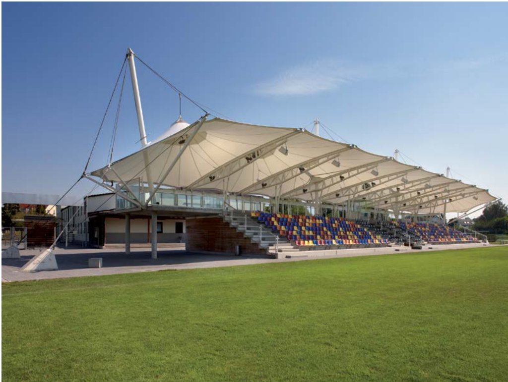
1 Membrane suspension with tension rods
