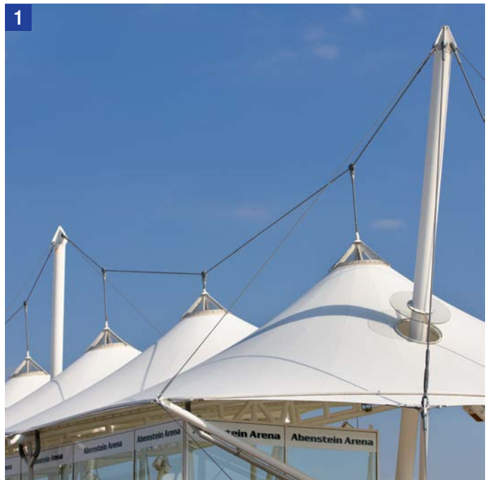
1 Membrane suspension with tension rods
