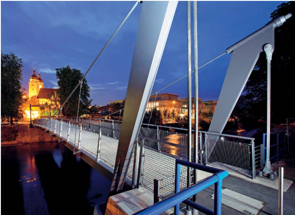
1 Anchorage of the hanger cable and suspension cables
