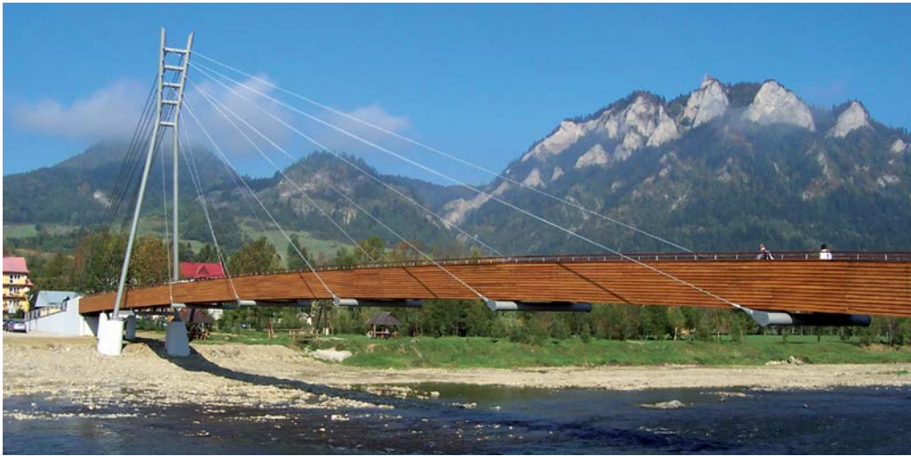
1 View along main pylon
