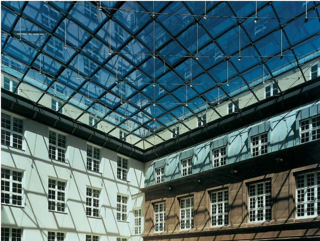
1 Stainless steel compression posts with supporting cables
