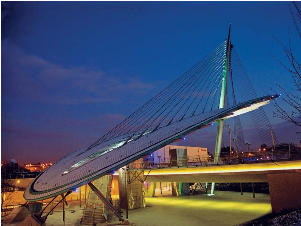
1 Pylon with harpe shaped staycables
