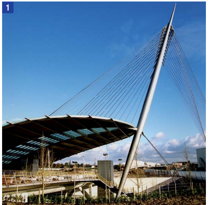
1 Pylon with harpe shaped staycables
