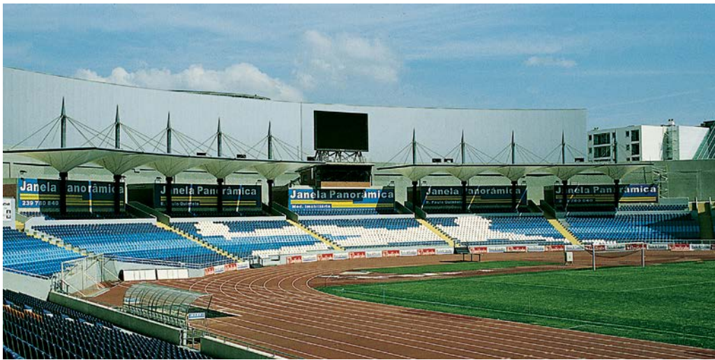
1 Suspensions of the membrane roof from the pylons
