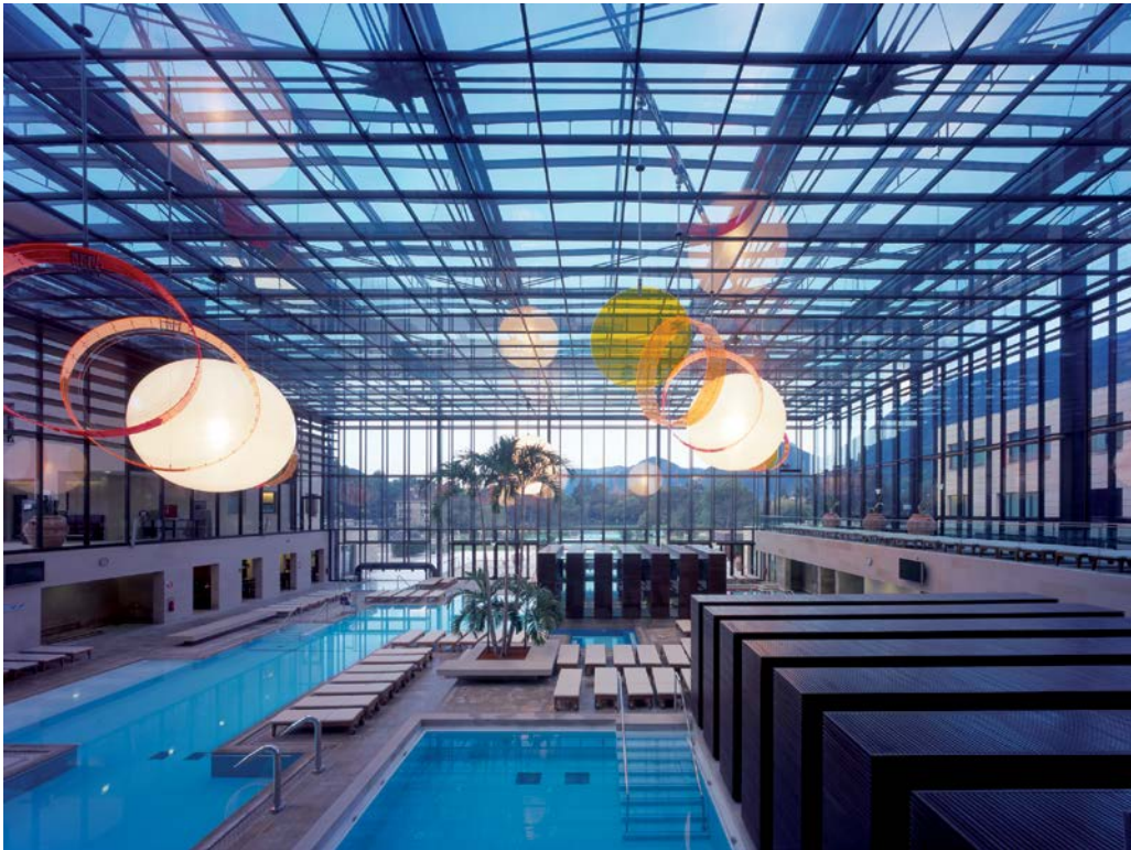
1 Truss system of the glass roof
