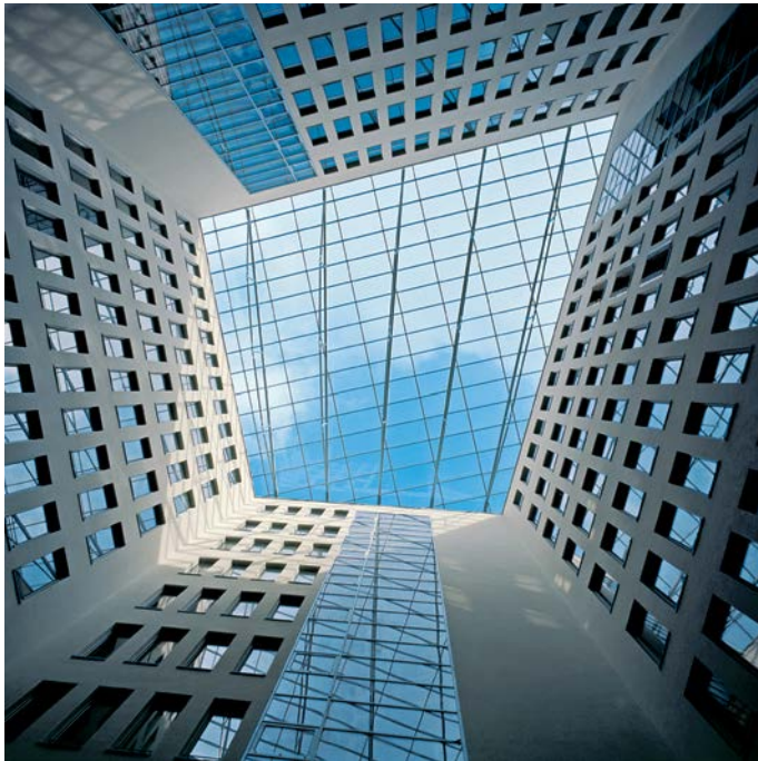
1 Truss system with tension and compression bars
