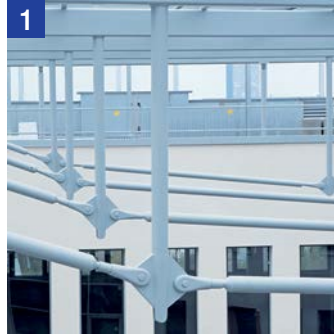
1 Truss system with tension and compression bars
