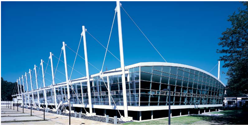
1 Pylons with pretensioned tension rod systems stabilised
