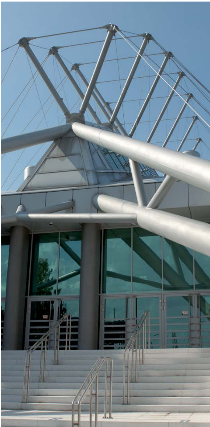
1 Exterior bearing system with tension rods
